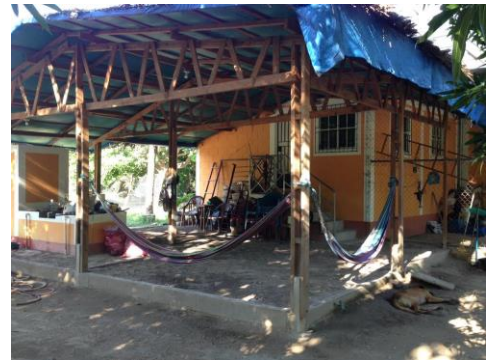
Building trusses and putting on roof over waiting area of Taura Medical Clinic, cost of clinic operation $600/month
