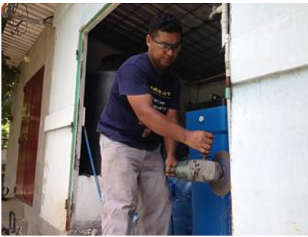
New doors on the water system building
