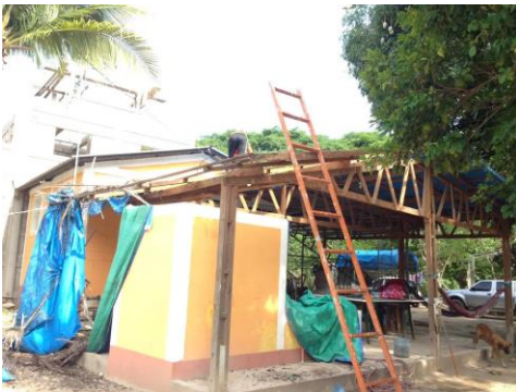
Building trusses and putting on roof over waiting area of Taura Medical Clinic, cost of clinic operation $600/month
